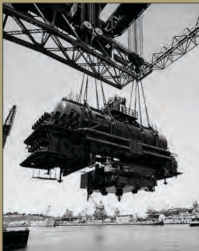
Preparation for the SEALAB project
