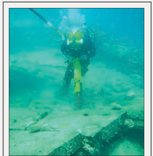
Equipment Operator 1 st Class Leroy Schnathorst is utilizing underwater hydraulic tool to break apart concrete sections for removal. (Photo by Petty Officer 2 nd Class Michael Price)
